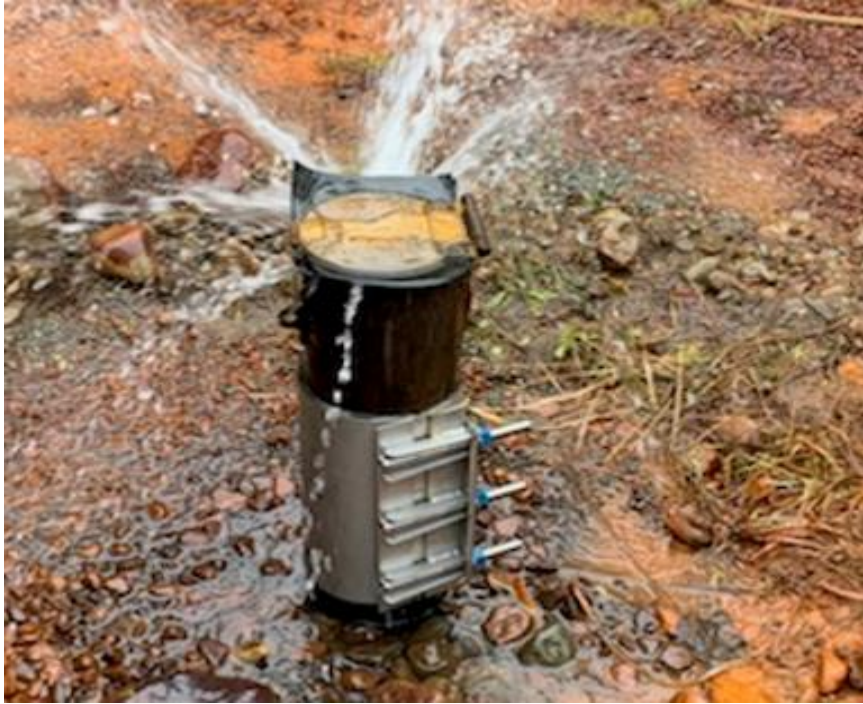
Figure 4: March 19, 2021 well capped and discharge reduced to about 1 L/s. Discharge still directed to the sump area. No surface expression to the river from the well. Well stopped discharging on May 13, 2021 when mine pool was reduced below 226 mASL.
